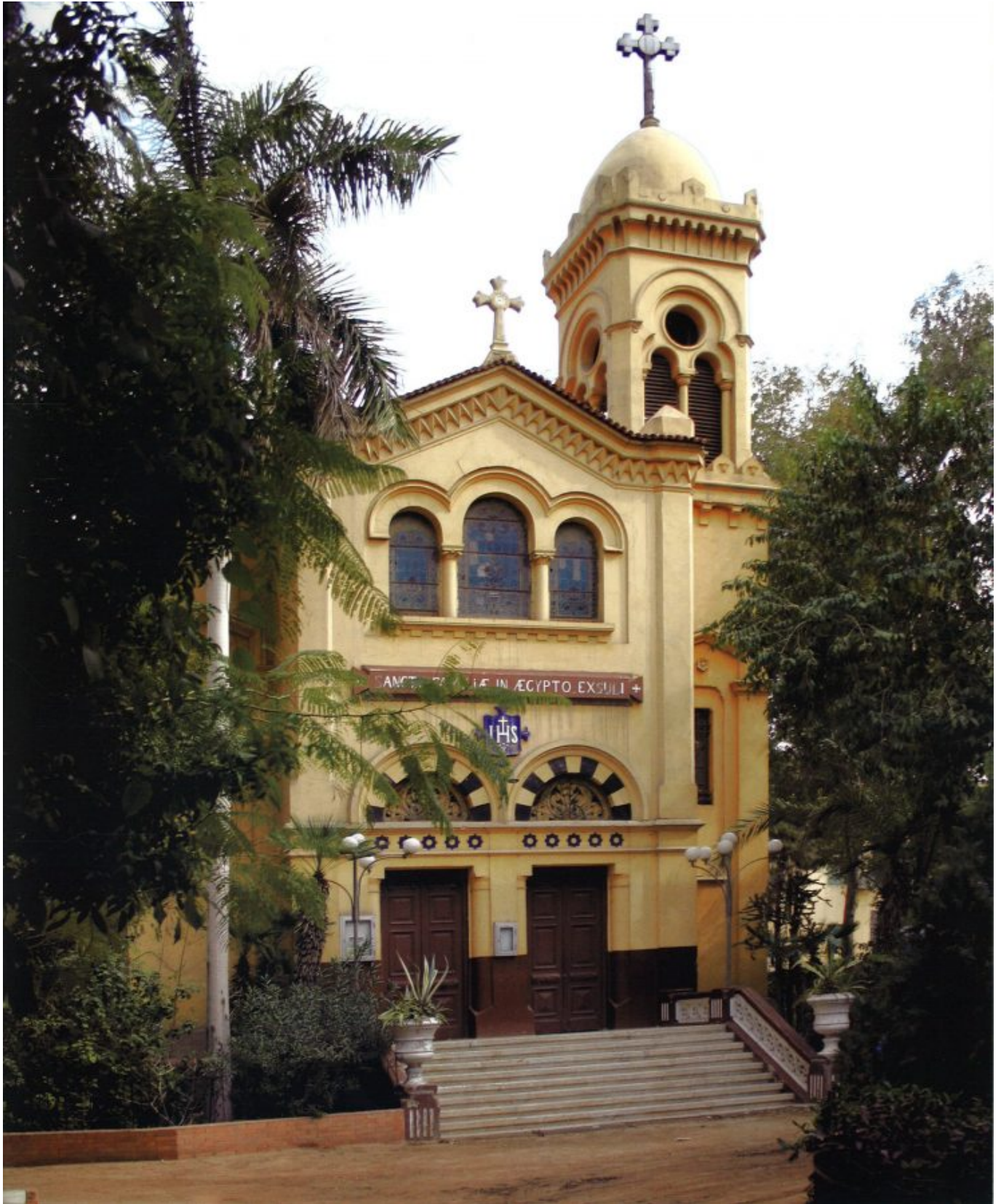
Exterior view of the Jesuits' Holy Family Church, Matariya.
